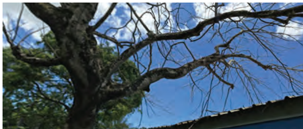
Figure 20: Example of a large dead tree with branches overhanging a classroom building.
