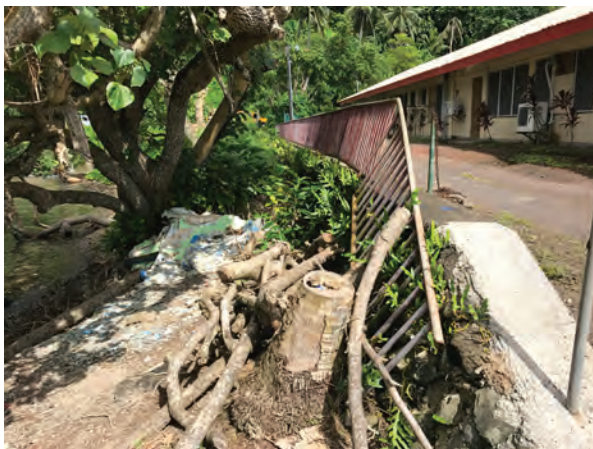
Figure 13: Dumping of trash and foreign debris should never be allowed on school grounds.
