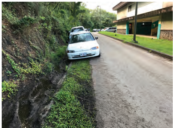
Figure 19: Vehicles parked within a drainage structure damages the planned function of the swale and causes storm water to backup and flood to other areas of campus. These parked cars are also blocking the fire access lane.
