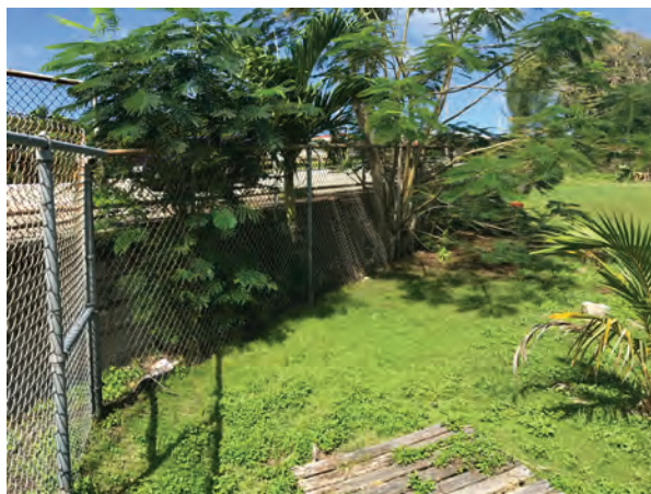
Figure 17: Trees growing along the fence also disrupt the drainage swale and should be removed.
