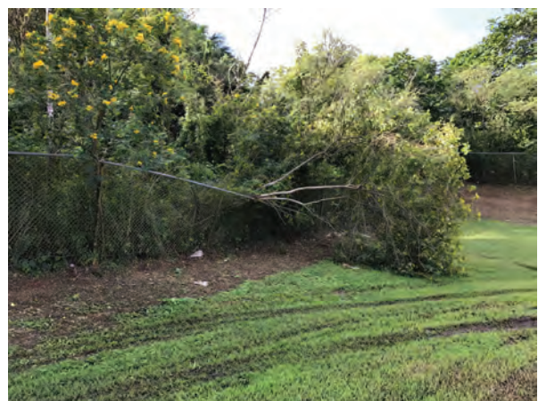
Figure 15: Fallen trees and overgrown vegetation has damaged section on perimeter chainlink fencing.
