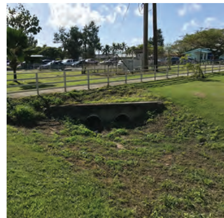
Figure 5: Drain Pipe Headwall
