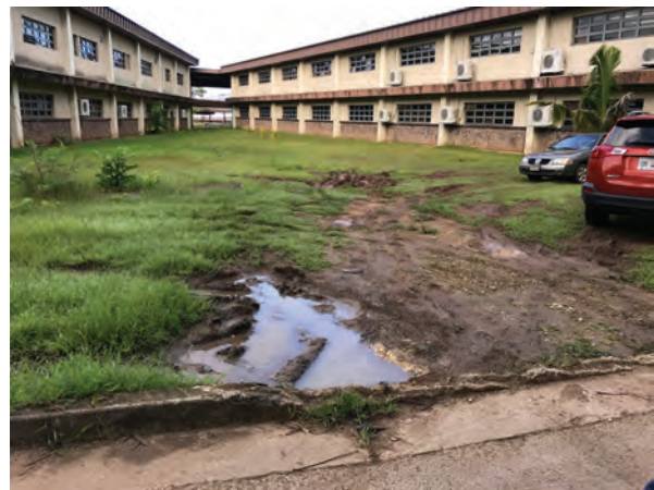
Figure 18: Vehicles parking on grassed areas damages the turf and creates potholes, which degrades site condition, causes erosion, and may create breeding habitat for mosquitoes.
